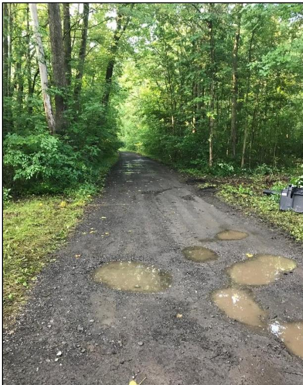
**Photograph 1.** View of the north-south gravel dirt road entering the project site. Slightly overgrown vegetation along the road. Numerous potholes along the road, filled with water following a rain event.
